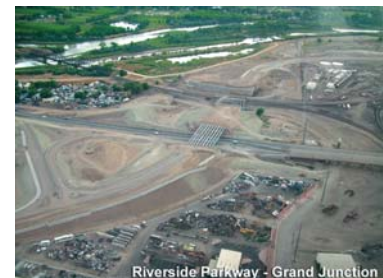
Riverside Parkway - Grand Junction
